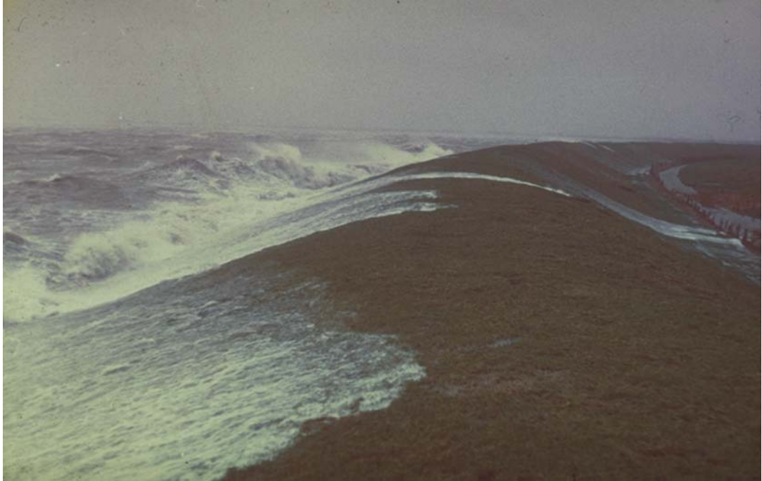
Fig. 5.23: Short crested waves resulting in wave run-up and wave overtopping (photo: ZITSCHER)
