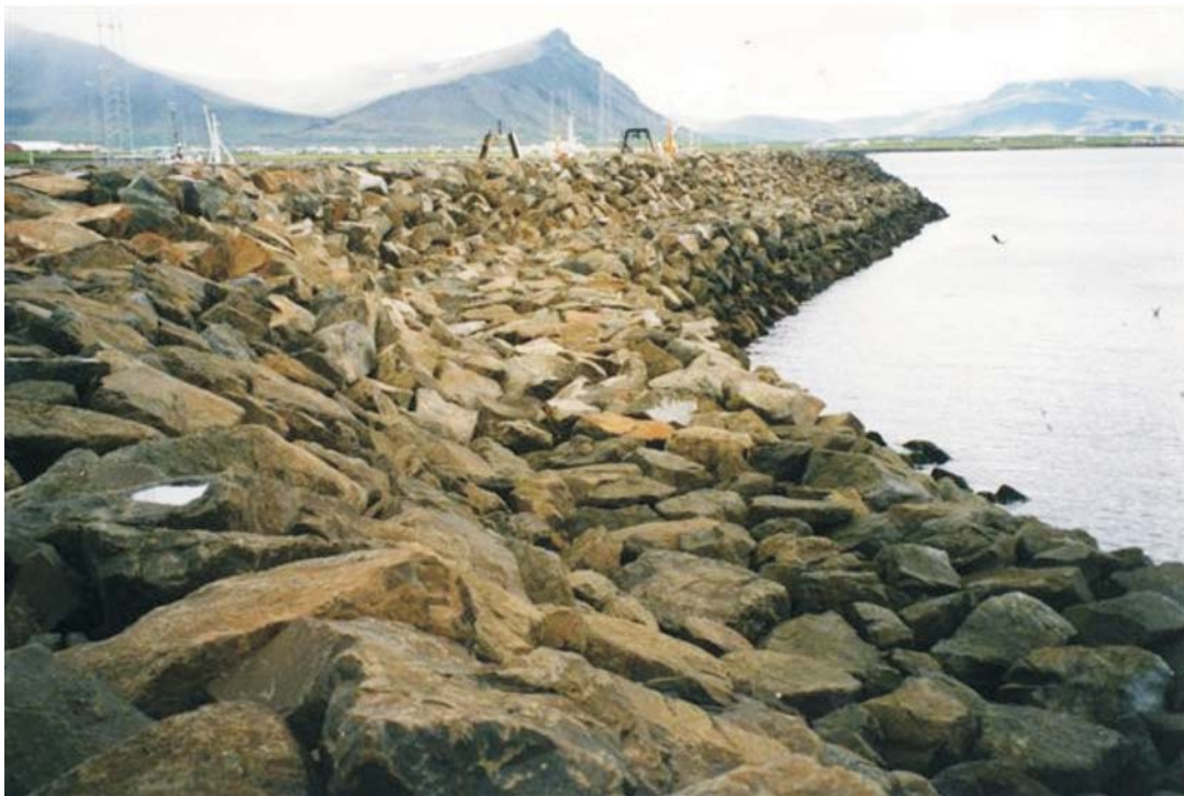
Fig. 6.7: Icelandic Berm breakwater
