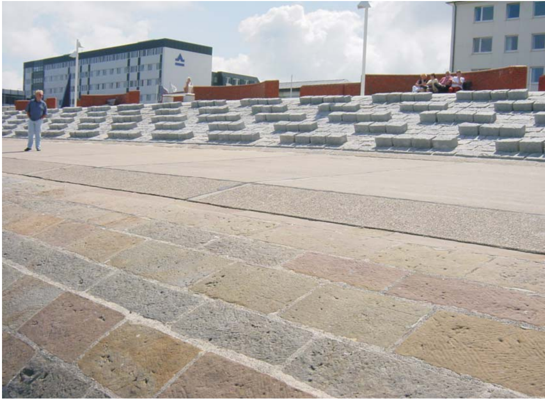
Fig. 5.19: Example for roughness elements (photo: SCHÜTTRUMPF)
