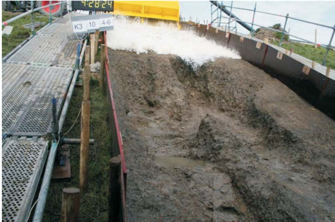
Fig. 3.2: Wave overtopping test on bare clay; result after 6 hours with 10 l/s per m width
