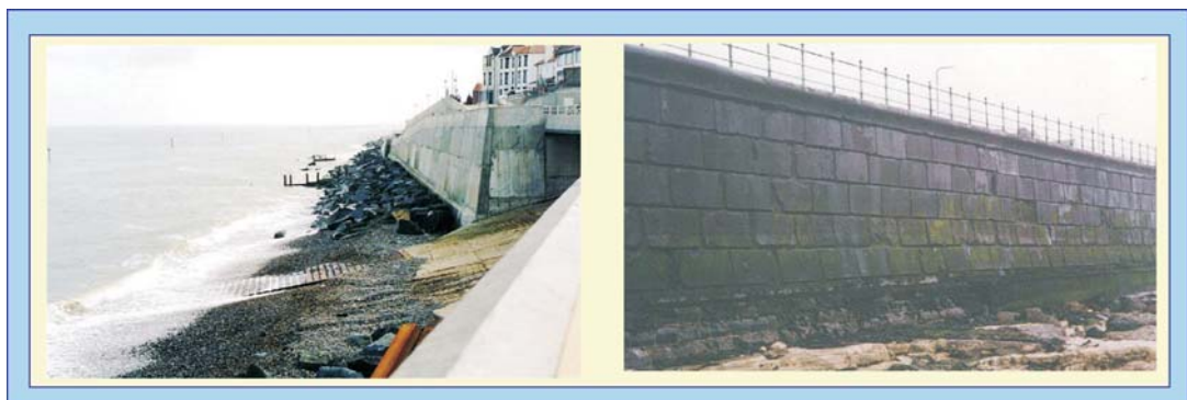
Fig. 7.2: Examples of vertical seawalls: (left) modern concrete wall and (right) older stone blockwork wall
