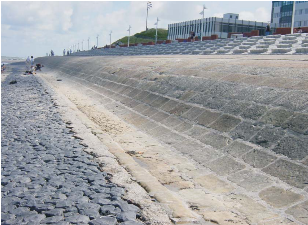
Fig. 5.17: Dike covered by natural bloc revetment (photo: SCHÜTTRUMPF)
